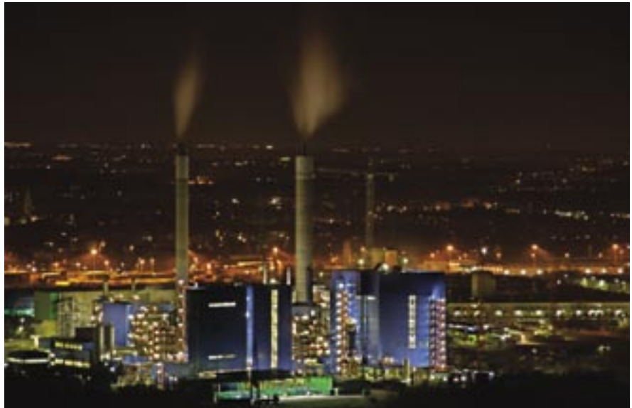
A waste incineration plant in Herten, Germany
